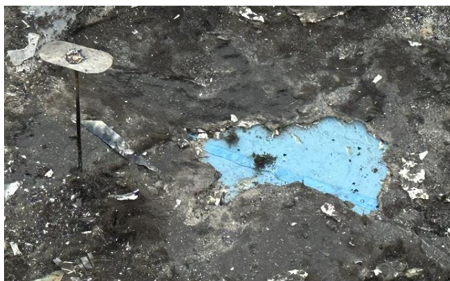
Figure 15 – From test 1. Intact vapour barrier observed below melted and charred EPS at the examined location.
