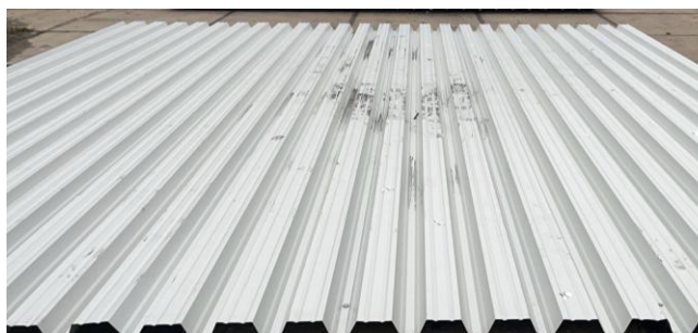
Figure 16 – From test 1. Trapezoidal steel deck after disassembly of the roof build-up. No residue from droplets formed by melted EPS noticed by the team at Troned test facility. From KIWA report.
