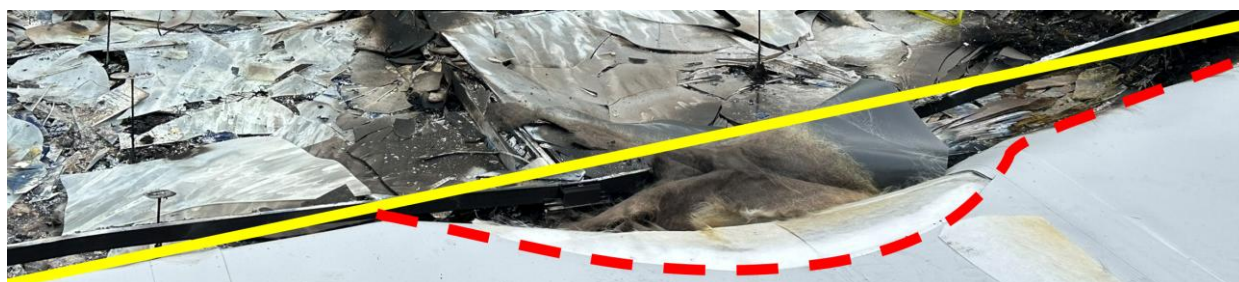
Figure 14 – From test 1. Yellow line indicates the original edge of the PV modules PV 4 and PV 3. The dotted red line marks the edge of melted EPS. Cutting of single-ply PVC membrane done by KIWA for the test report during inspection of roof damage.
