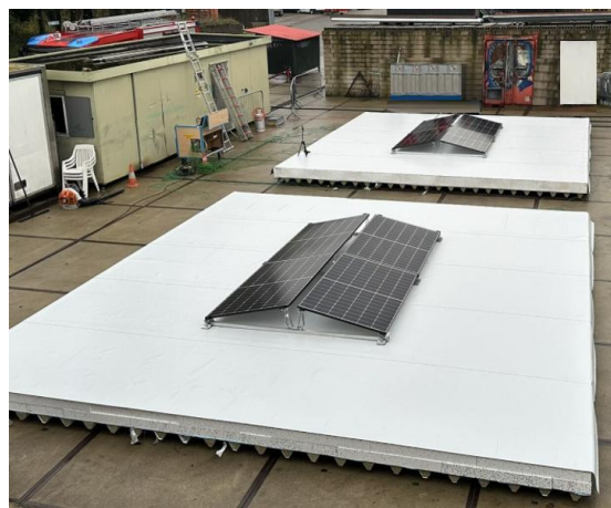
Figure 1 - Aerial view of test 1 and test 2 (closest) in October 2024 at the test area.
